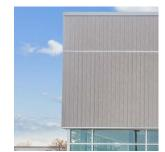
4. FIBER CEMENT BOARD NICHIHA LATURA V-GROOVE OR EQUIVALENT
