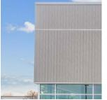
4. FIBER CEMENT BOARD NICHIHA LATURA V-GROOVE OR EQUIVALENT
